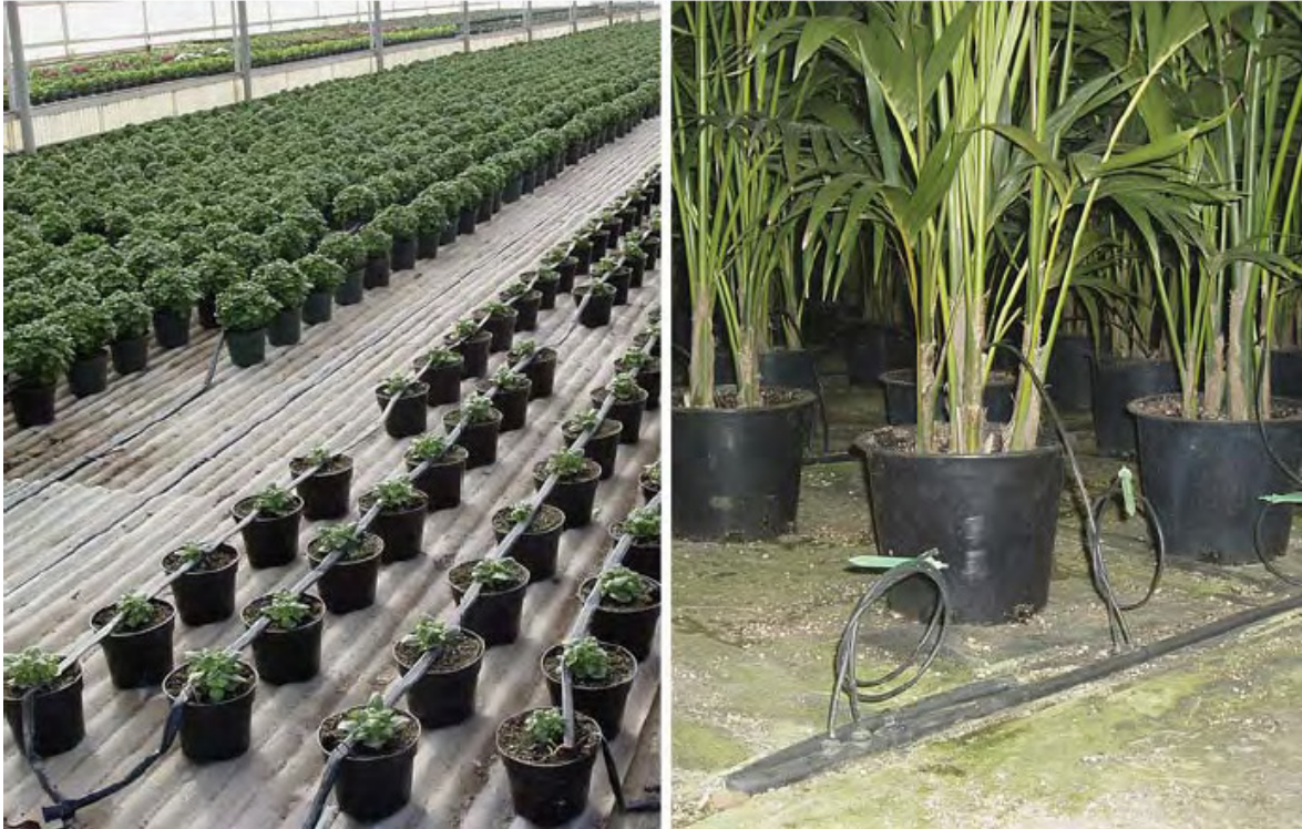
Figure 5-3. Drip tapes, left, and microirrigation stakes, right, are low-volume irrigation systems. (Source: Mangiafico, 2010)
